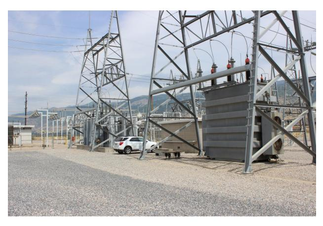
138 KV Substation 75 MVA Transformer (left) and 62.5 MVA Transformer (right).
