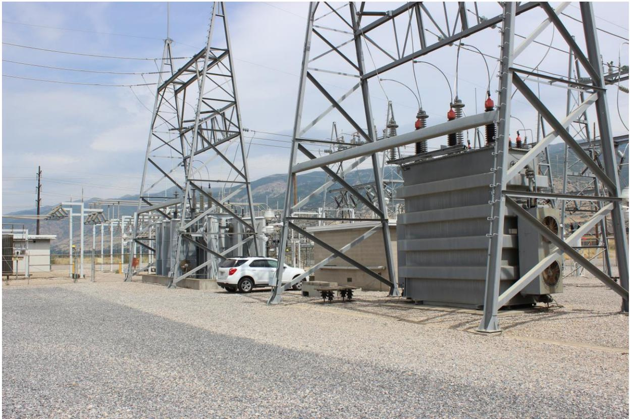
138 KV Substation 75 MVA Transformer (left) and 62.5 MVA Transformer (right).
