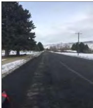
STREET VIEW LOOKING NORTH
