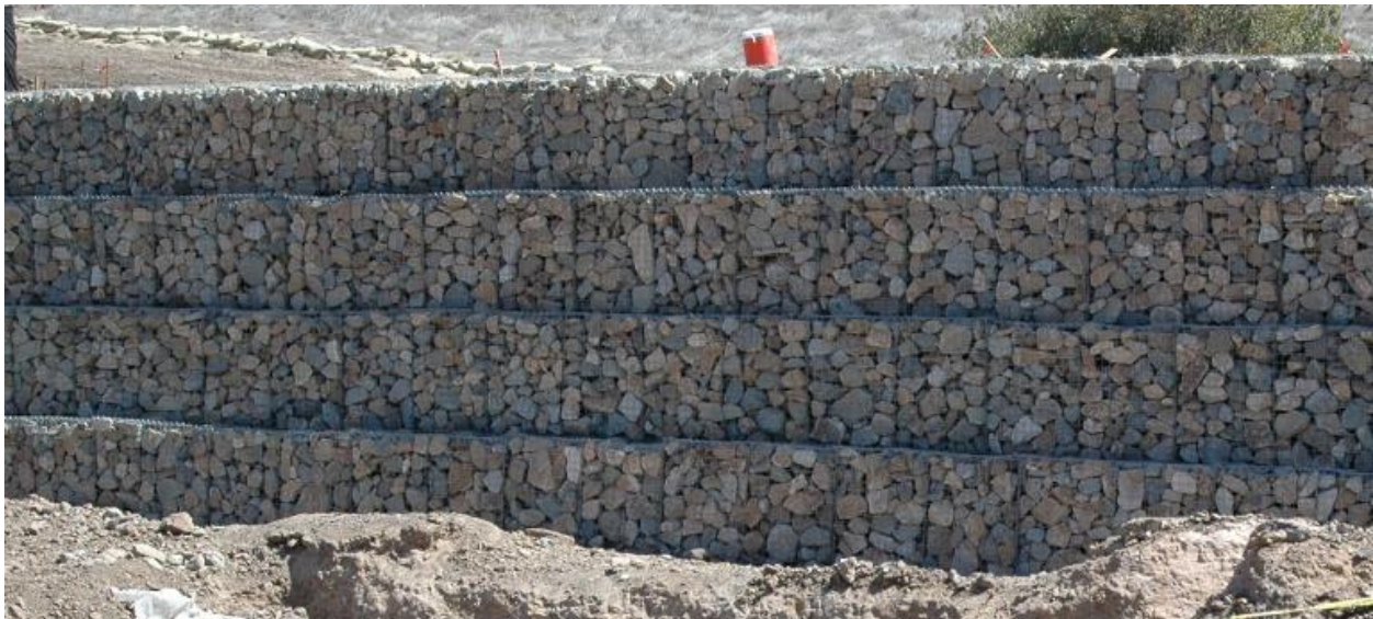
Figure 2 Example Photo of Gabion Wall Construction
