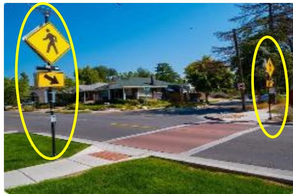
Figure 4 Rectangular Rapid Flashing Beacon (RRFB) Installation
