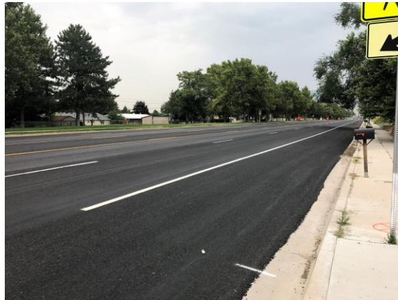
Microsurfacing work along US-89 from Eagle Ridge Drive to the I-15 connection is complete.
